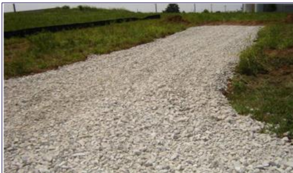
Figure 8.1: Temporary access track
