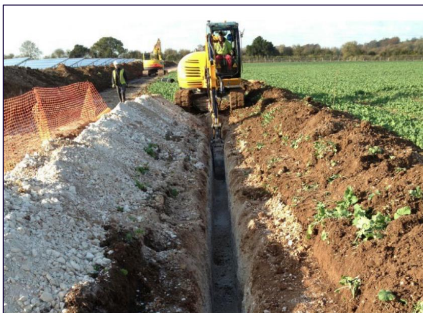
Figure 6.1: Cable trenching, showing topsoil stripped and set to one side, with subsoil placed on the other side ready for reinstatement (image courtesy of British Solar Renewables)
